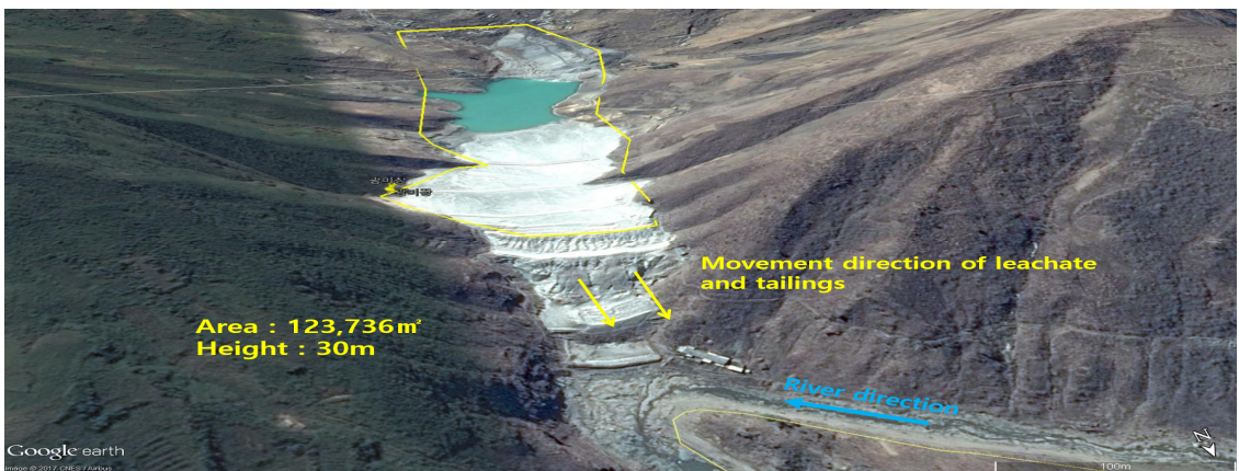
Fig. 4. The tailing dam of Holdong gold mine.
