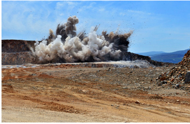
(b) Charging and blasting operation
