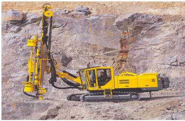
(a) Drilling operation
