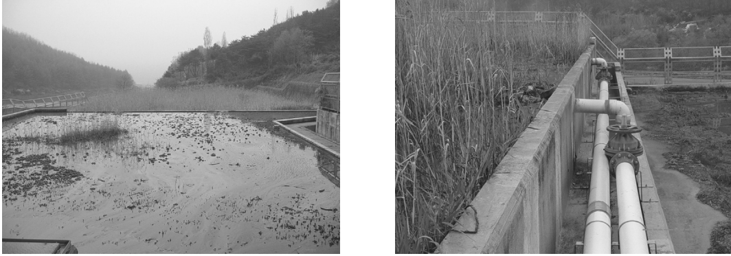
Fig. 2. Overview of the constructed wetland at Dalsung mine.
