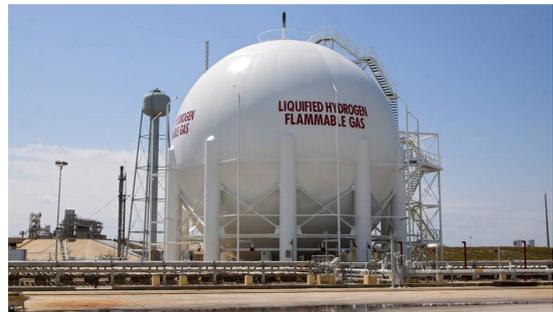
(b) Cryogenic spherical vessel of NASA, USA (NASA website)
